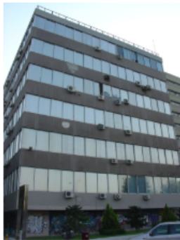
Surveying Engineering building 5 th floor
